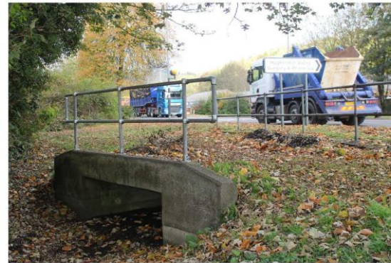
PHOTO 2. Side view SED 1 – Culvert Crossing
